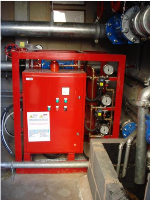
The SD200 has been designed to overcome the problem of low main's pressure. The intelligent system continuously monitors its situation and adapts its response accordingly. It maintains the pressure in the Sprinkler system at the designed level while preventing damage to the town's main.
